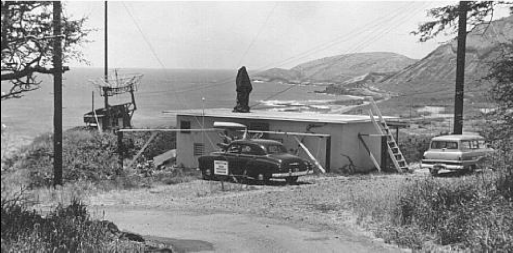
The University of Hawai'i Solar Observatory at Makapu'u Point, Oahu, 1967. The solar radio noise 10-ft dish is at the left. The heliostat mirror is at the left end of the building.
