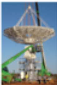
Assembly of the first ASKAP antenna node under construction. Credit: CSIRO pathfinder CSIRO
