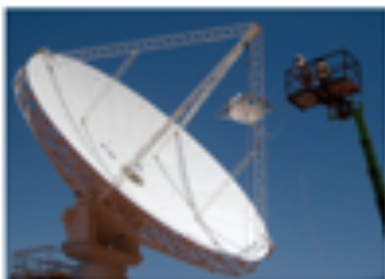
Lifting the antenna plant into feed housing. Credit: CSIRO pathfinder CSIRO
